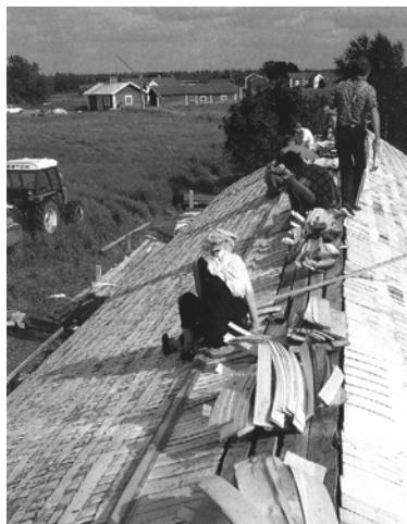
Picture 4: Making of shingle roof
