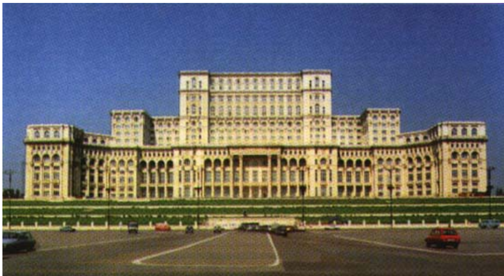
Fig. 12. Proof of the intrusion of politics in the life of the city, dull neo-classical solemnity, 3,107 rooms - 742 of them are used as offices
