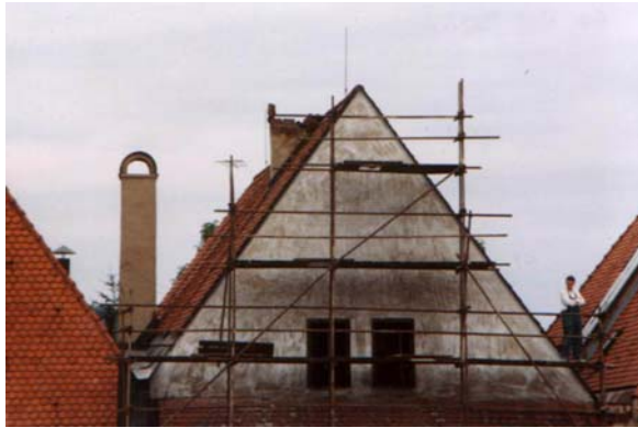
Repairing of the plaster of main facade was finished without repairing of deteriorated top of the chimney. House No. 38, Tawn Hall square, Bardejov before and after repairing of main façade.
