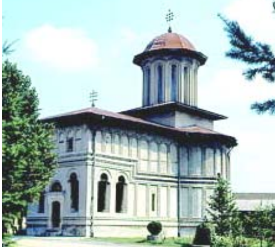
Figure 2 : Church of Plumbuita Monastery-1647
