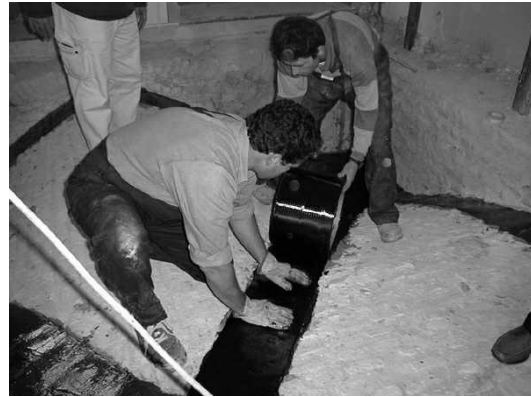
FIGURE 19: The fixing operation at the extrados of the vault
