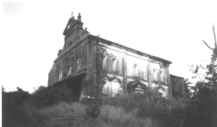
Figure 1: View of the Capella De Monte from the South West.
