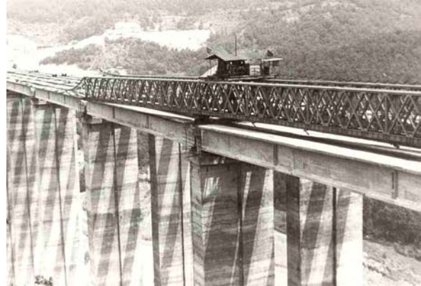
Fig.33. Assembling of bridge girders.
