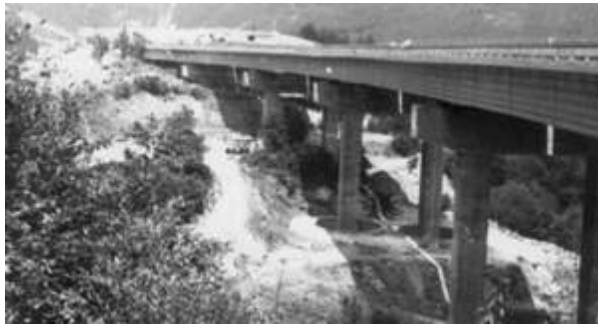
Fig.37. Six spans continuous beam
