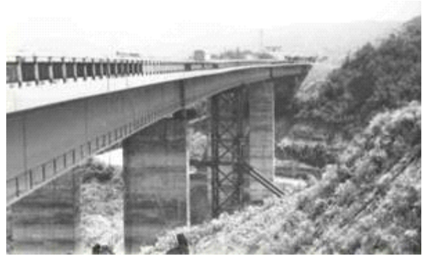
Fig.38. Three spans continuous beam
