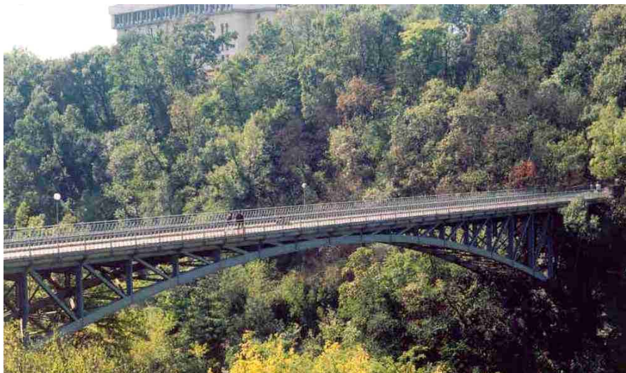
Fig. 34. "Stambolov" Bridge in V. Tarnovo
