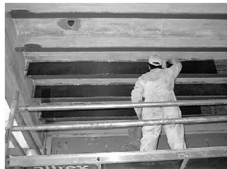
Figure 5.1: External reinforcements using steel plates and CFRP (Library, Leuven, (B))
