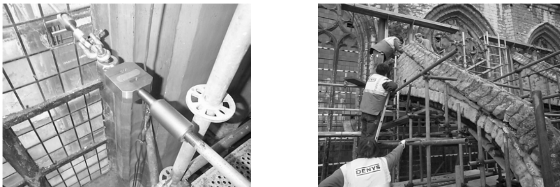
Figure 3.1: load cell in truss and removal of flying-buttress
