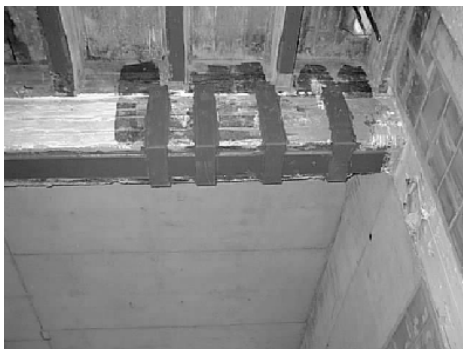
Figure 5.1: External reinforcements using steel plates and CFRP (Library, Leuven, (B))
