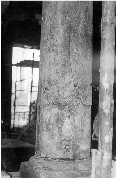
Fig. 2 Cracked column [5].
