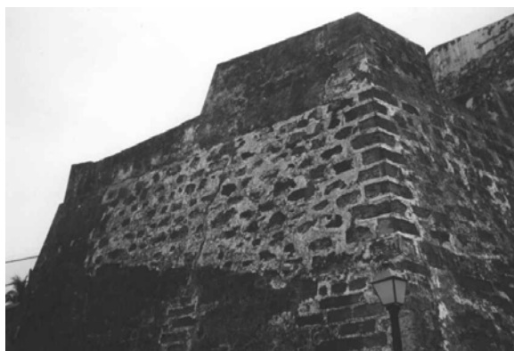
Fig. 4 – View of the walls of S. Juan, Puerto Rico
