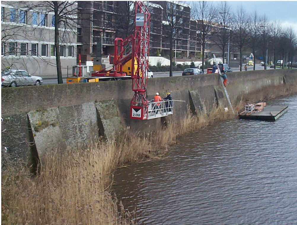
Fig. 11: The historic rampart of 's Hertogenbosch is geo-electrically measured.
