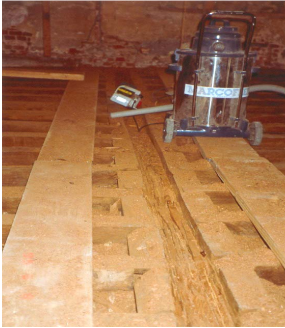
Fig. 15: A large groove is milled out of the wooden beam and reinforced with steel bars and filled with epoxy mortar
