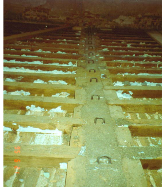
Fig. 15: A large groove is milled out of the wooden beam and reinforced with steel bars and filled with epoxy mortar
