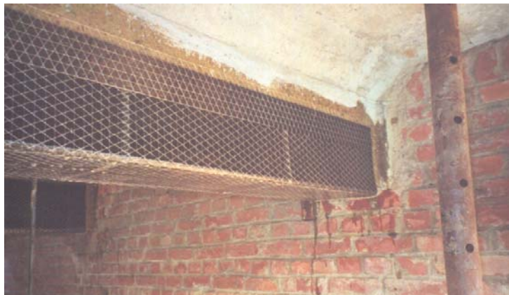
Fig. 13: External reinforcements using CFRP (Tienen (B))
