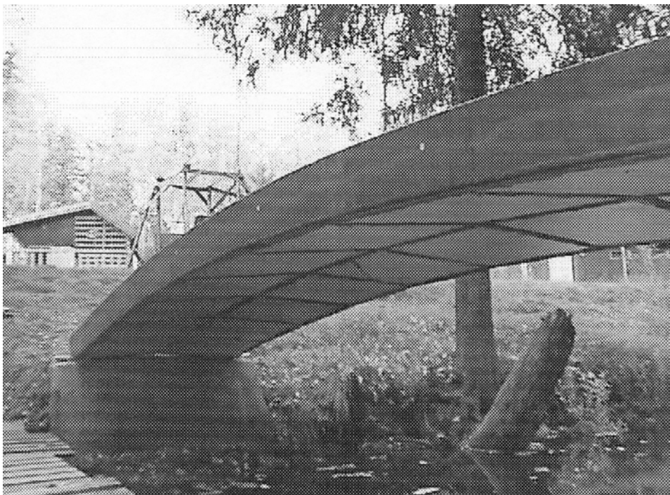
Jorma A. Eskola and Raimo Tikka, 1999, University of Oulu, Department of Architecture. Span 6,5 meters and weight 240 kilos.
