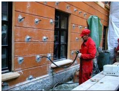
Figure 6: Grouting of stone masonry
